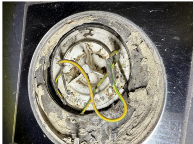
Sluk under servant-stor hybel
