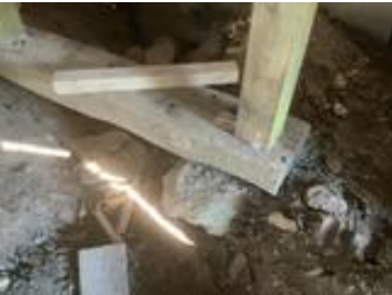
Ufullstendig fundamentering.
