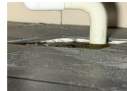
Sluk under badekar- begrenset adkomst.
