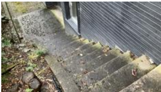
Trapp i betong.
