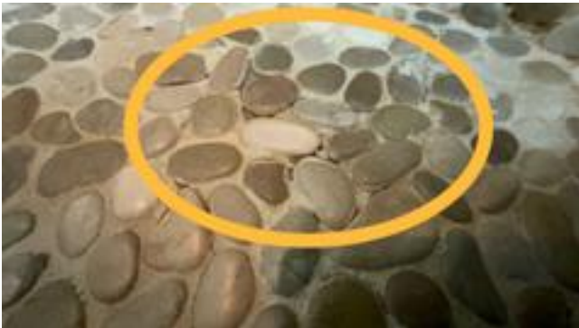
Sprekker i betongfuger
