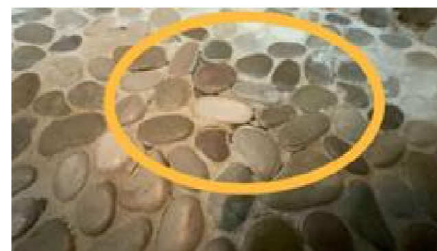
Sprekker i betongfuger
