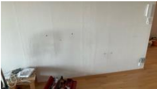
Falming/plugger i vegg.
